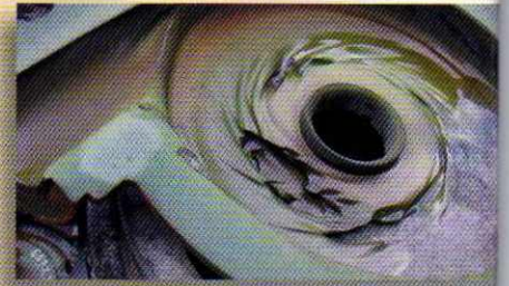
Daily repair routine – can no longer be repaired with traditional technologies available on site. No responsible wants to be in such a situation any more . . .
